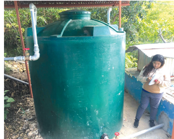
A water filtration system for a safe water source of the barangay . The water can be safely consumed with the same value as the commercially available purified water.
