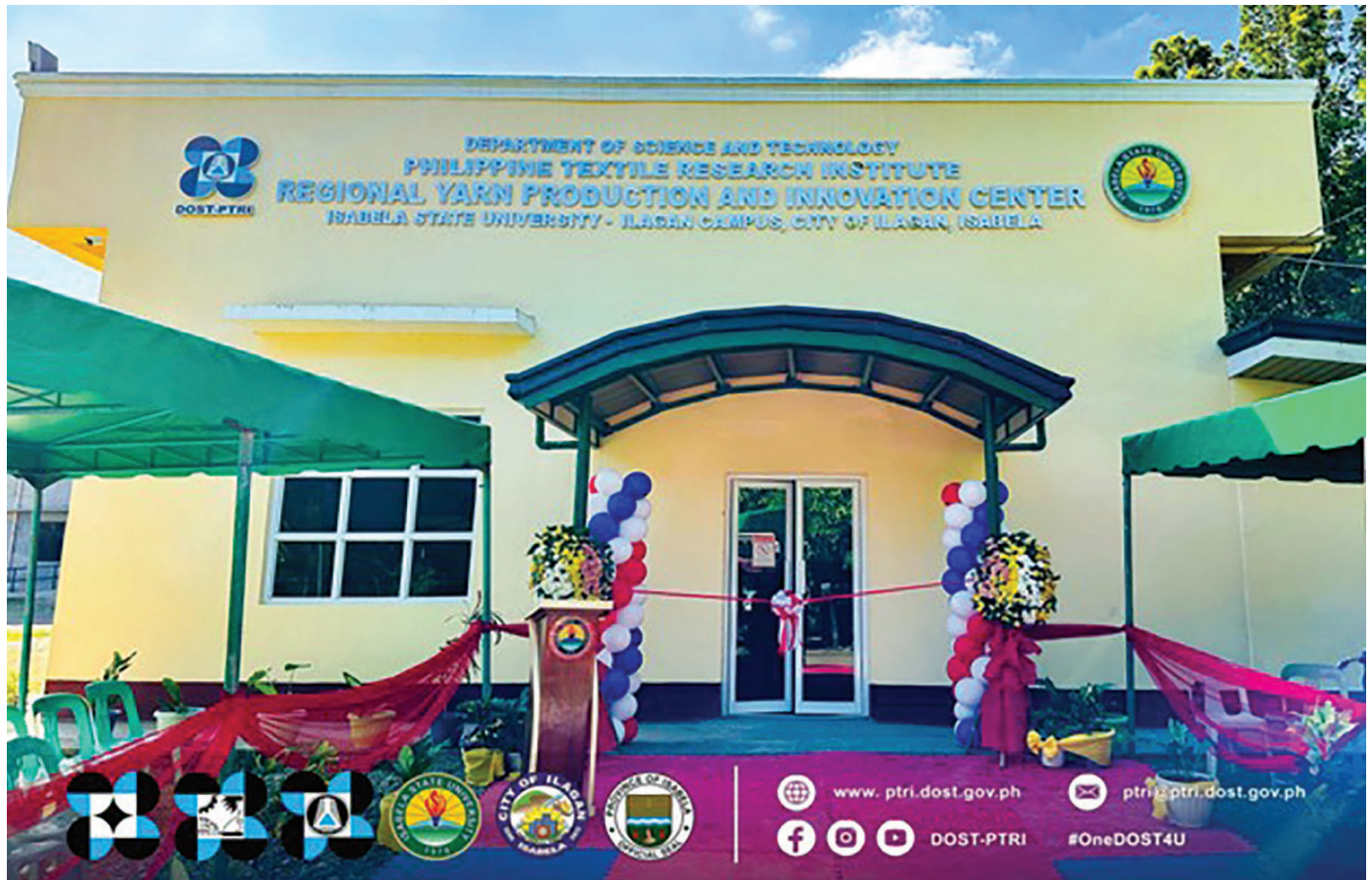
1st Regional Yarn Production and Innovation Center in Isabela.
